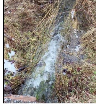
Roadside Ditch - Catchment
