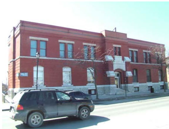
Cobourg Police Services Building
